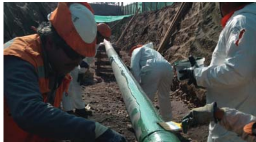
Sonacol staff applying the Protal 7200.
