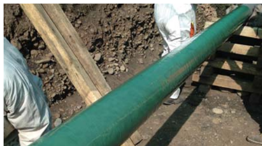
Protal 7200 applied at very high film thickness.
