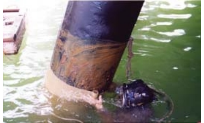
Denso Marine Piling Tape being applied underwater.
