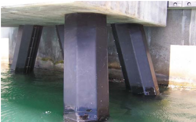
US Navy Ford Island Bridge - Pearl Harbor, HI
